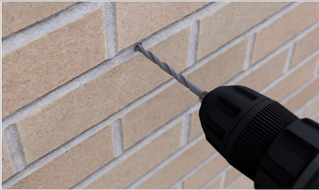
Drill -slightly inclined upwards- an 8 mm hole in the joint for the pin.
