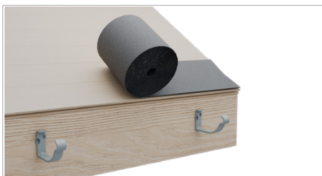
Lay a strip of fascia sheet underlay.
